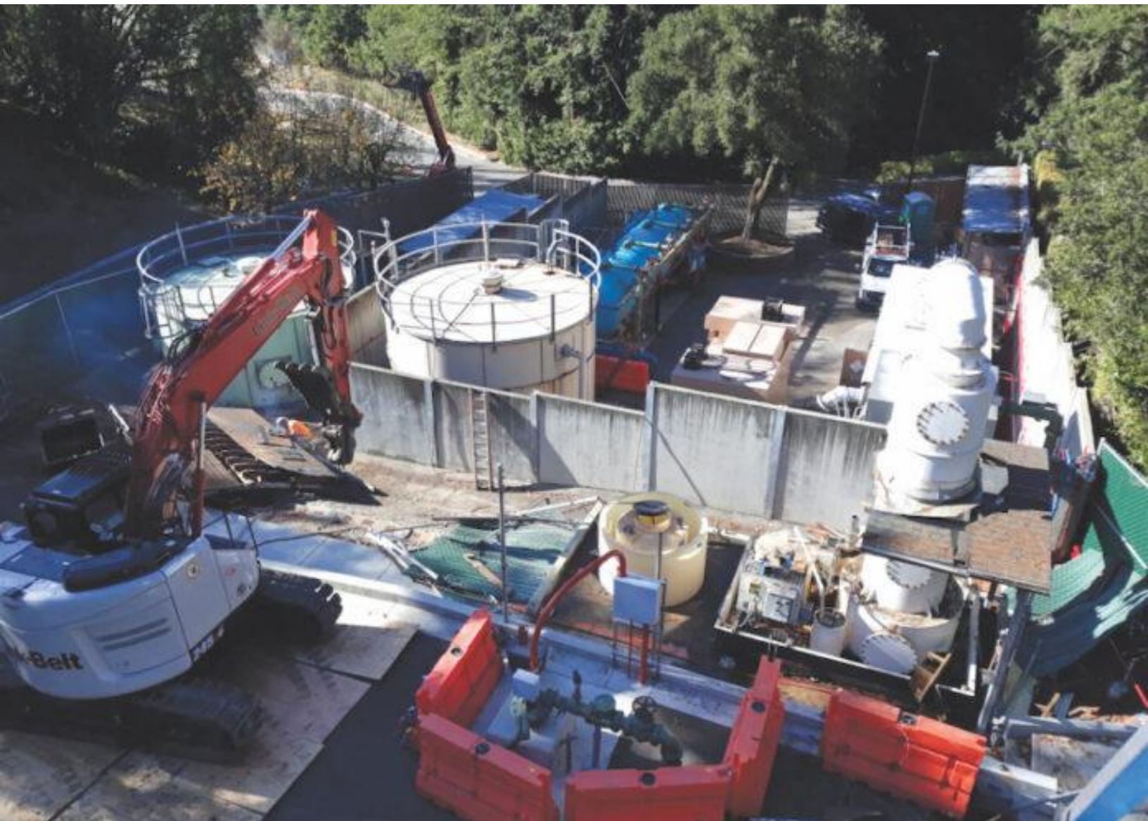
Figure 5-12: SVWD Water Treatment Plant Upgrade
