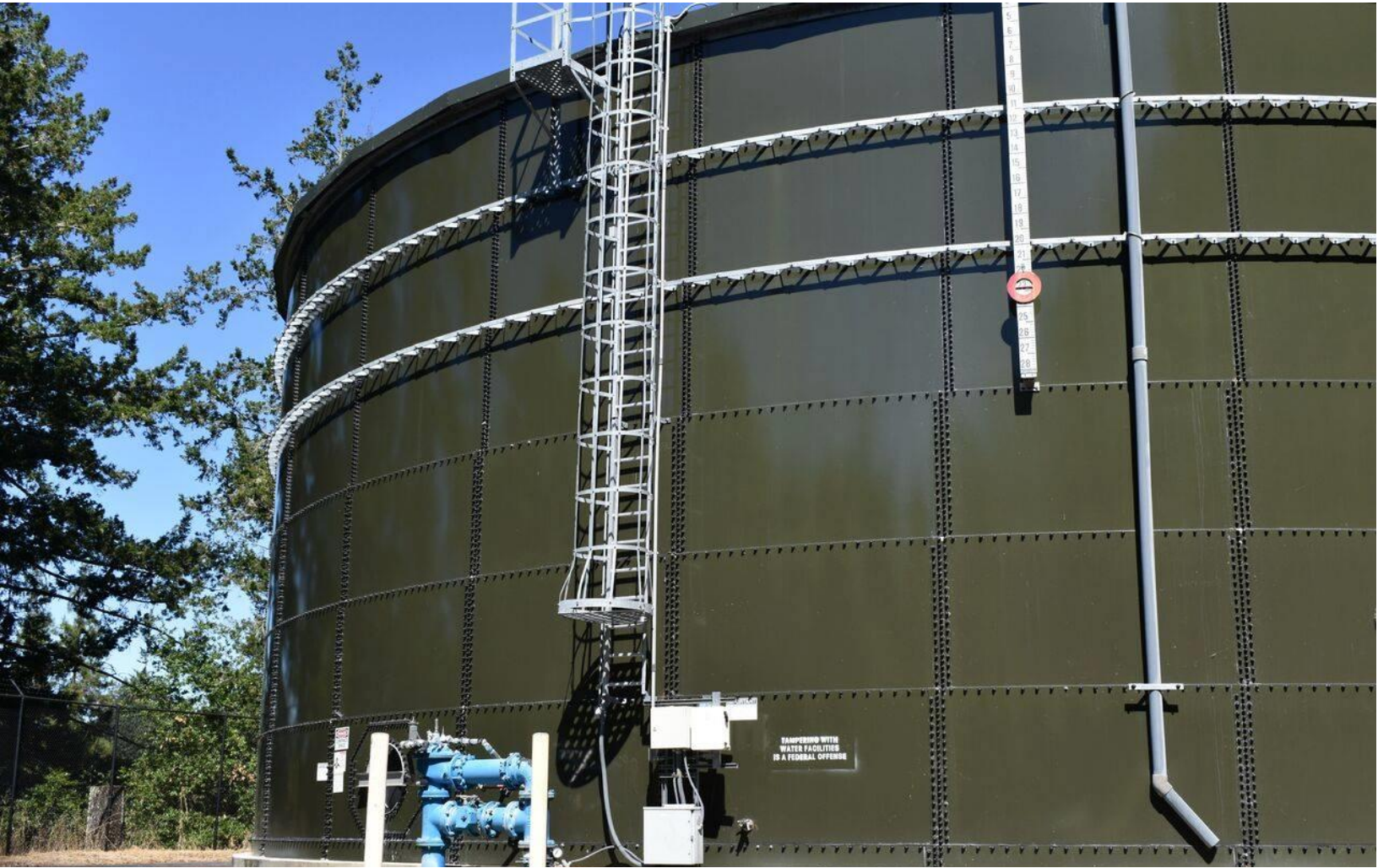
Figure 5-13: Bethany Tank Rehabilitation Project
